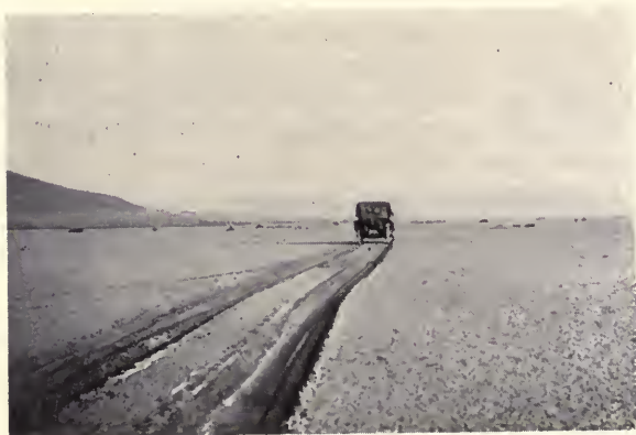
On the Lincoln Highway across Nevada there are several of these mud flats. When dry they afford excellent going, but when wet become absolutely impassable for motor traffic and have caused great hardships and delay to transcontinental motor tourists. Extensive improvements, now under way, will make for comfortable travel through this region
